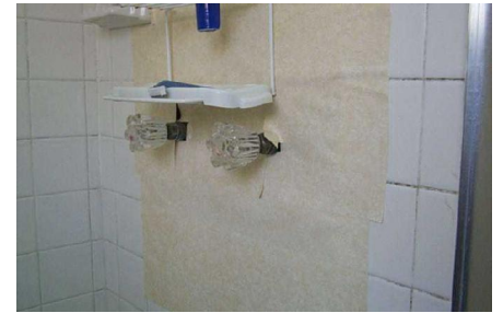
Figure 3. Shelf paper being used to hold shower tiles in place.
