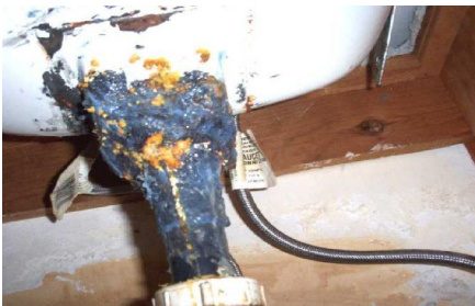
Figure 4. Silicone sealant being used as plumbing repair.
